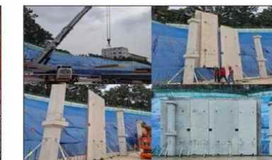
Suwon Jangnan Underground Parking Lot
