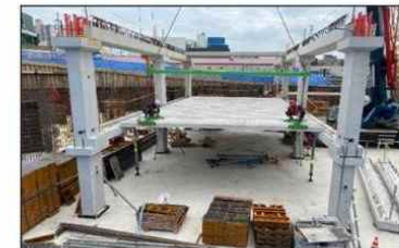
Underground parking lot PC construction site
