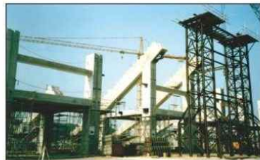
PC Columns, Beams, Girders and Stand of Ulsan World Cup Stadium, Korea
