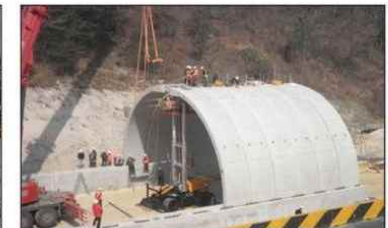
Guangming Tunnel Construction Site.
