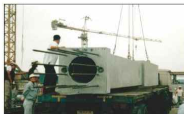
PC Columns, Beams, Girders and Stand of Ulsan World Cup Stadium, Korea
