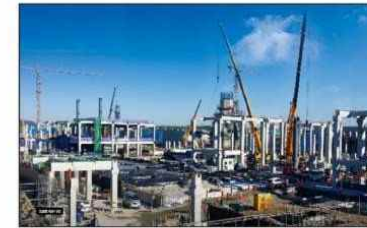
Incheon Airport Terminal 2 PC structure construction site
